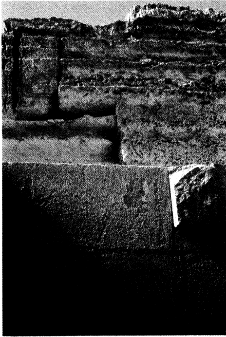
Figure 11: Limestone blocks in the north face of the Great Pyramid of Khufu, in Egypt. Weathering of this stone over several thousands of years has failed to mar the excellence of fit of the blocks; only minor surficial pitting has occurred under the arid conditions involved.
